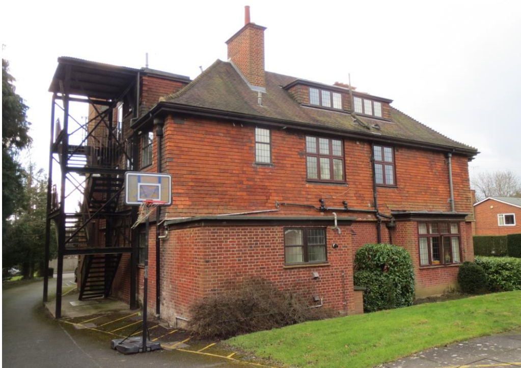
Plate 5: Northern and eastern elevations of Aldis Hall and later fire escape.
