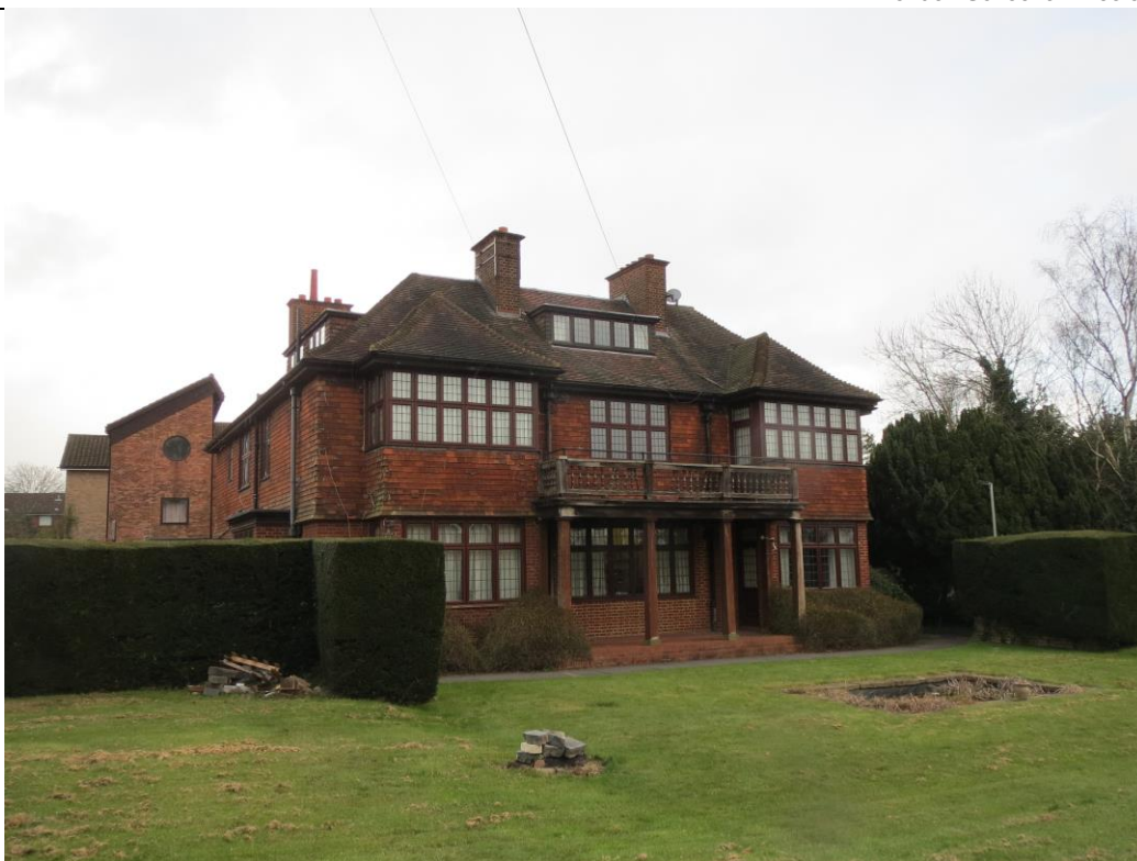
Plate 3: West front of Aldis Hall, looking south east
