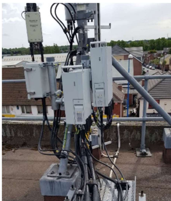
Source: Blackheath Telephone Exchange – 5G antenna support apparatus
