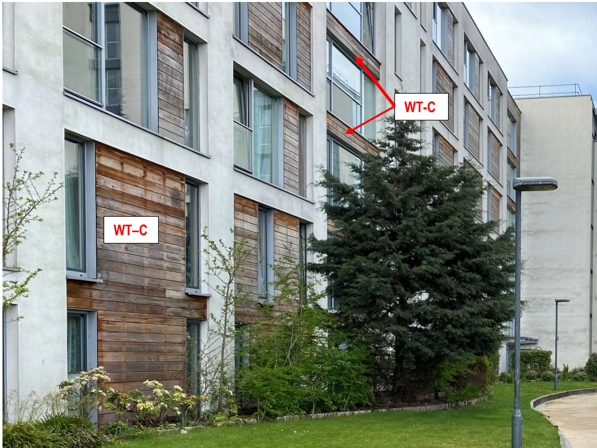
Fig. 22 – Photo above shows the North Elevation of Block E and the different configurations of the timber rainscreen (Wall Type C);
