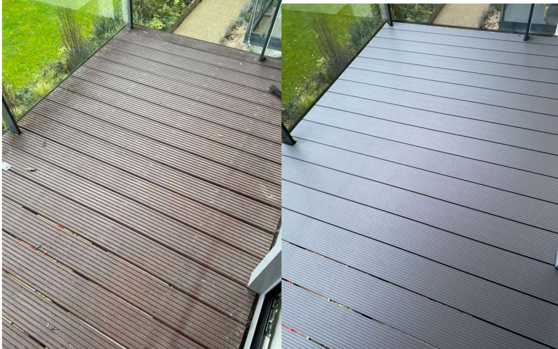
Fig. 15 – Second Example of a completed balcony decking replacement; the left-hand side photo shows the original timber decking balcony, the right-hand side photo shows the same balcony and the completed aluminium decking replacement.
