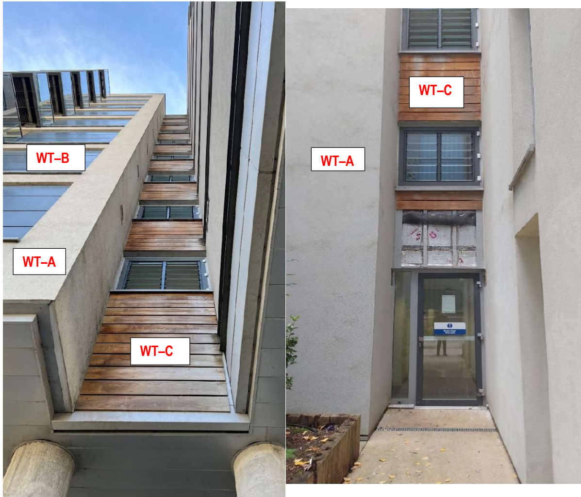
Fig. 21 – Photos above show the North (left hand side) and South (right hand side, above) short elevations and the AOV windows – the configuration is similar across all Blocks (A – E)
