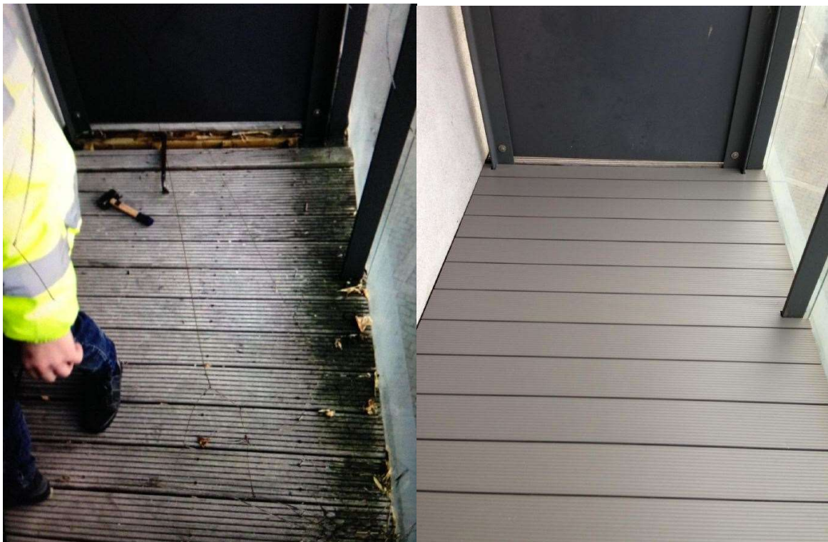
Fig. 16 – Third Example of a completed balcony decking replacement; the left-hand side photo shows the original timber decking balcony, the right-hand side photo shows the same balcony and the completed aluminium decking replacement.
