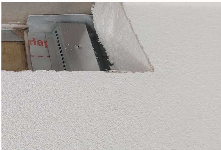
Fig. 23 – Photo above illustrates the Existing EWI Render System (WT-A); photo was taken following intrusive inspections.
