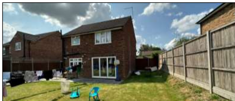
Rear Elevation of the Appeal Property
