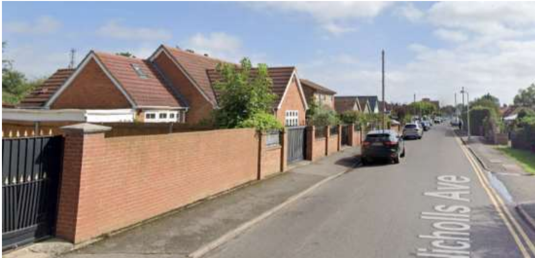
Olive Tree House restricts views of the appeal site on approach from the west
