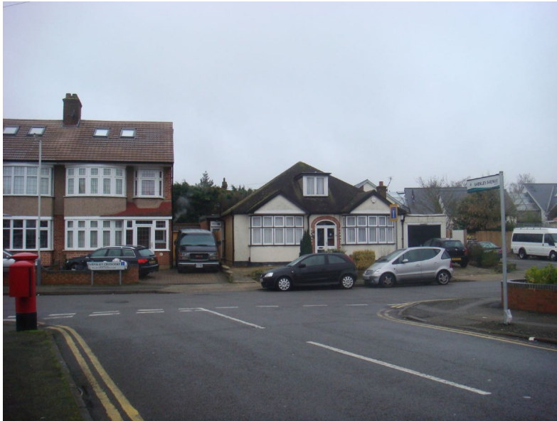
35 Eversley Crescent showing the recently completed hip to gable to the adjoining house
