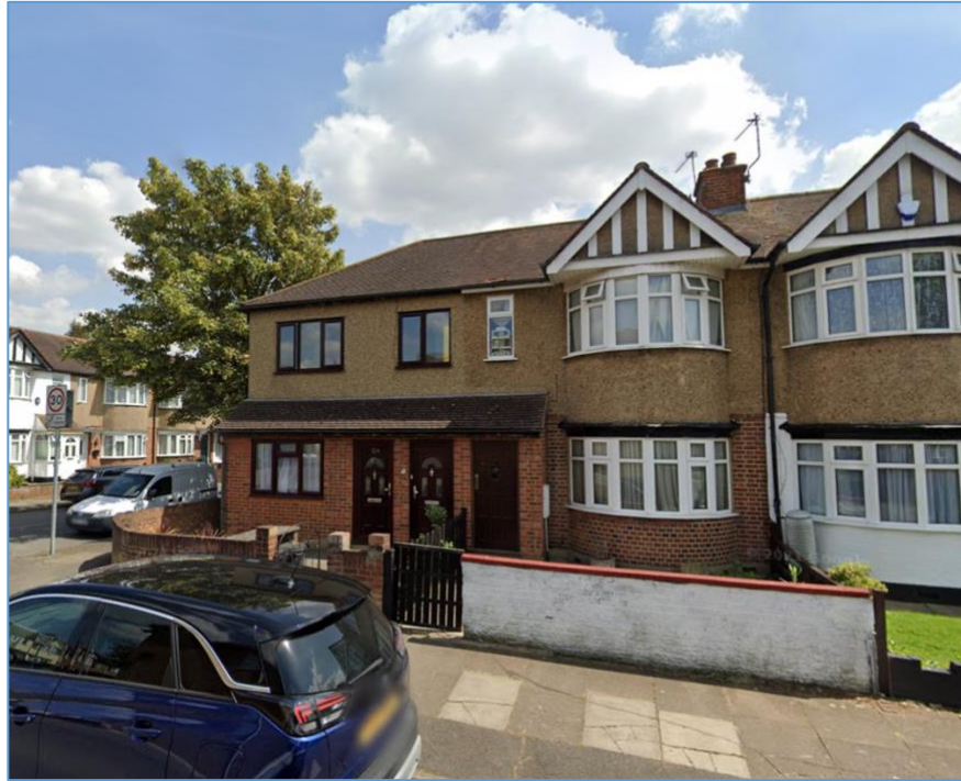
Figure 5: Two-storey side extension at 32 Sidmouth Drive.
