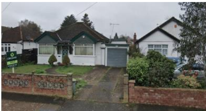
No 20 Halford Road prior to redesign
