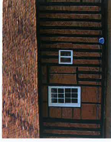
Fig 5.18 Old Mill House- timber framed barn with stained weather boarding
