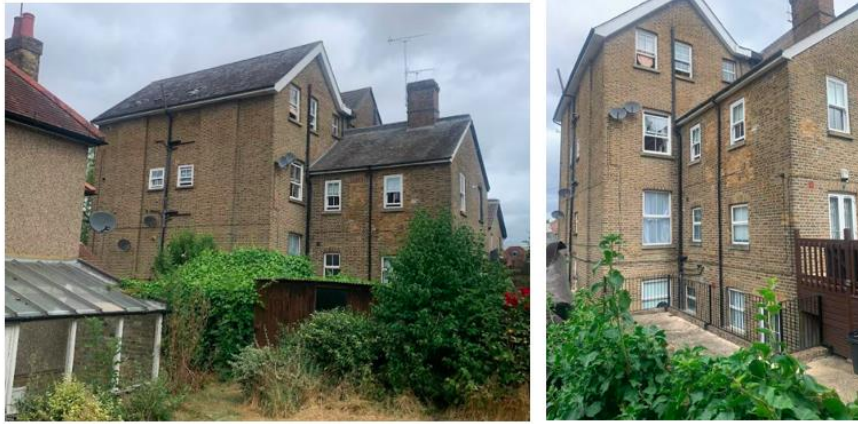
Views of the side and rear elevations of no.74 Harefield Road, showing number and nature of side windows evident
