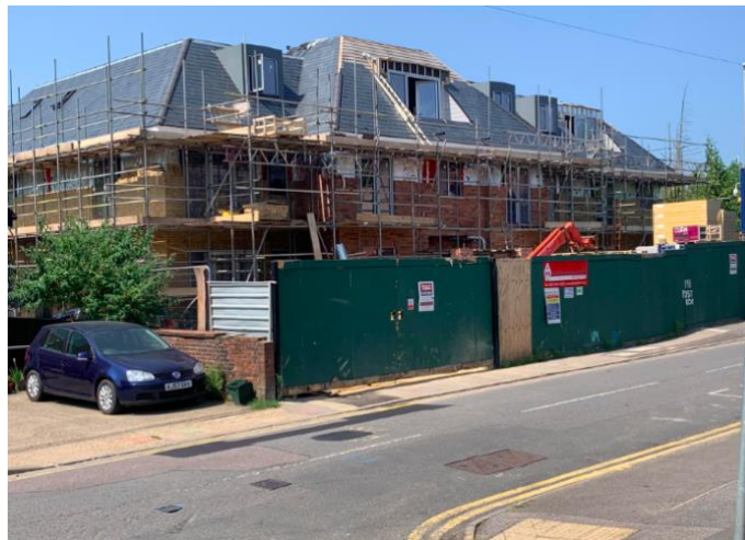
Development of the former Abrook Arms PH
