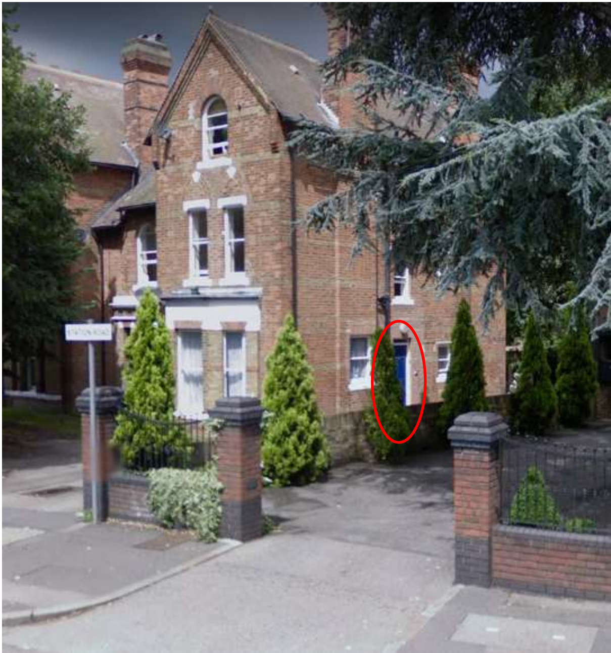
Photo 3: 169 Station Road has a side entrance door.
