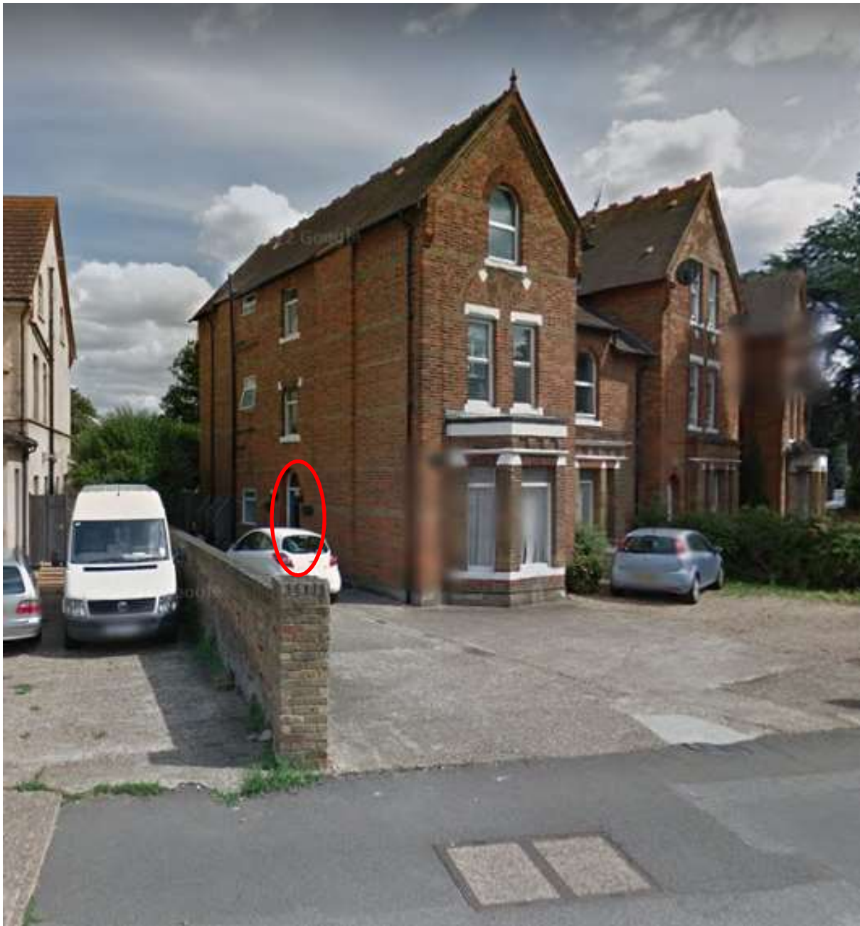
Photos 4: 165 Station Road has a side entrance door.
