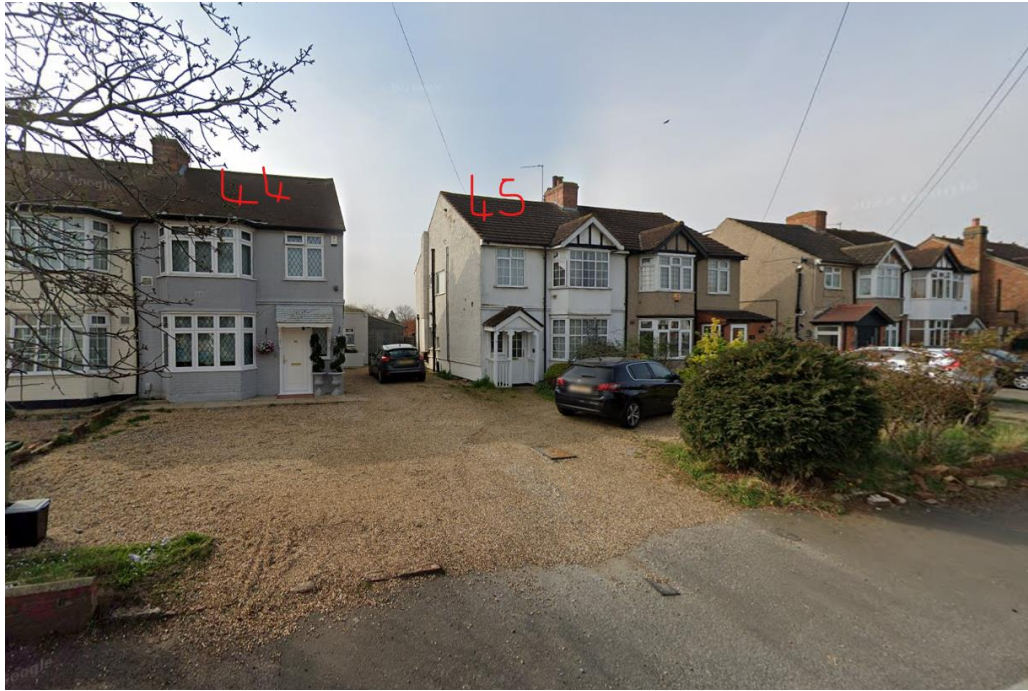
Figure 4 - May 2022 street scene view of appeal site
