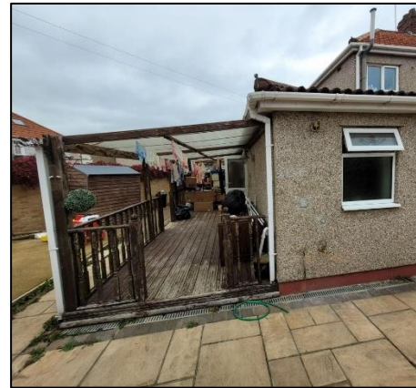
Existing Canopy – Rear Elevation
