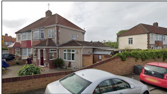
High Side Boundary Wall
