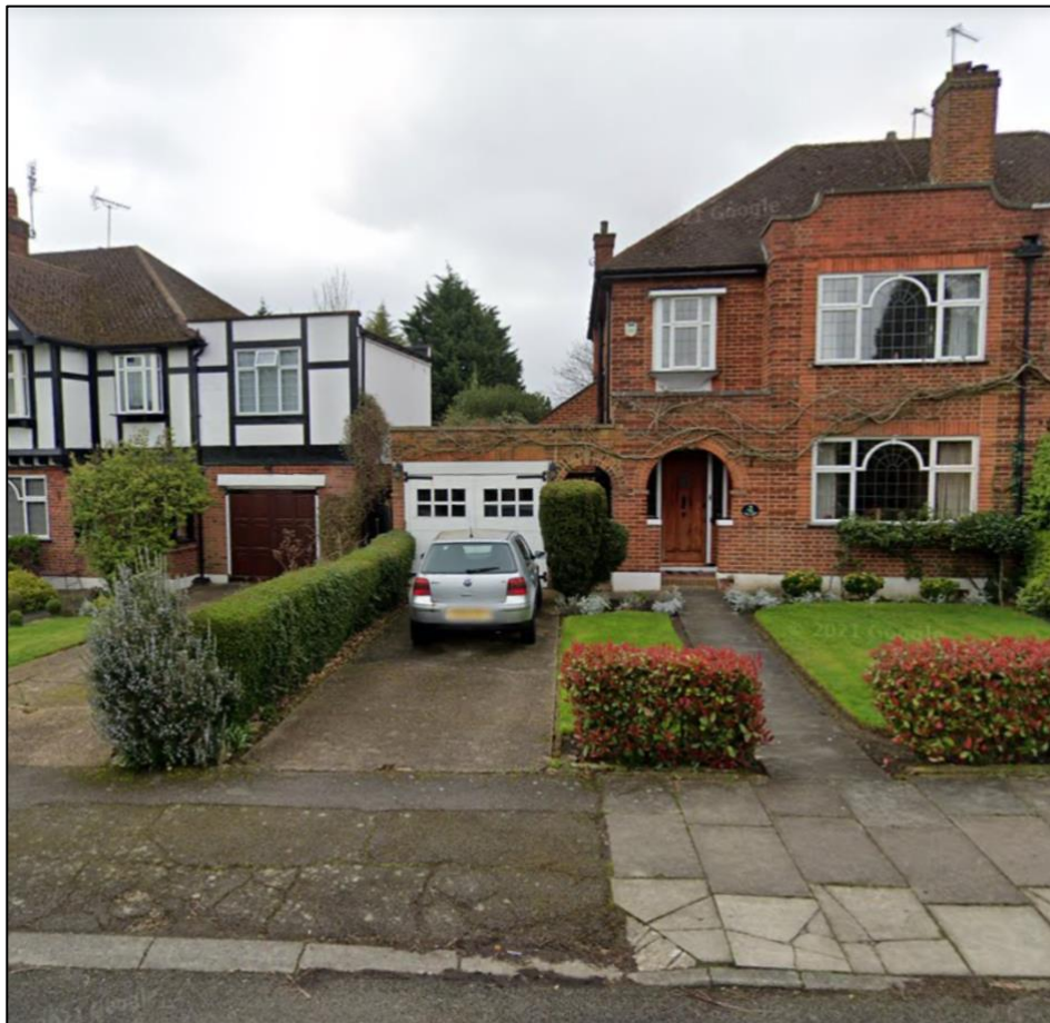
Figure 2: Numbers 26 and 28 St Lawrence Drive, prior to the recent development
