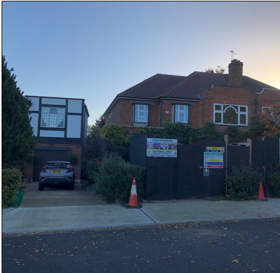
Figure 3: Numbers 26 and 28 St Lawrence Drive, following the recent development
