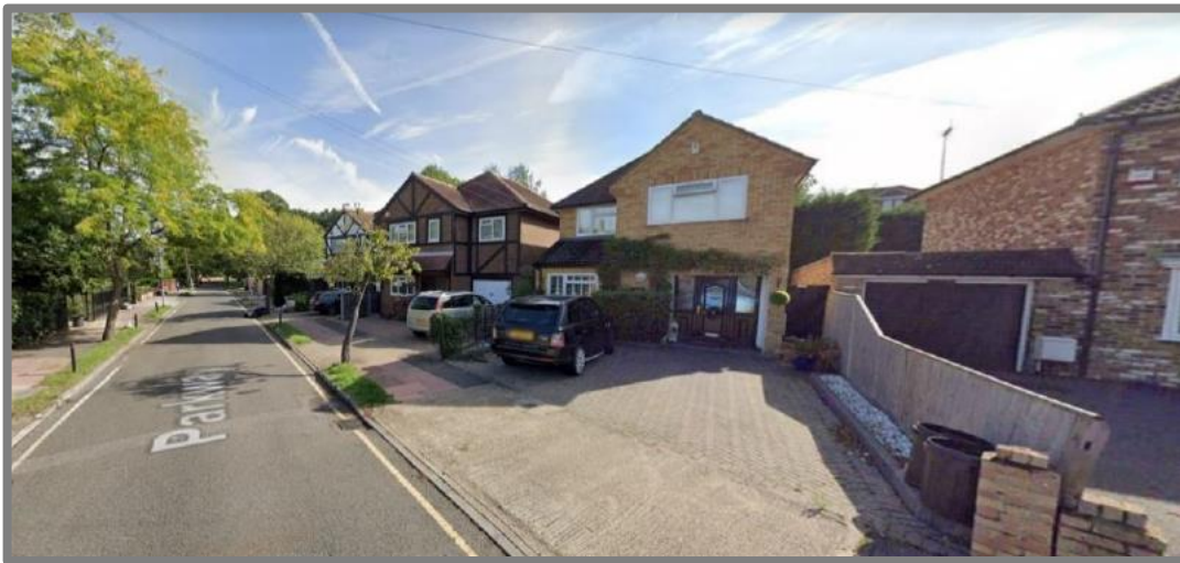
Figure 2: Properties along Parkway
