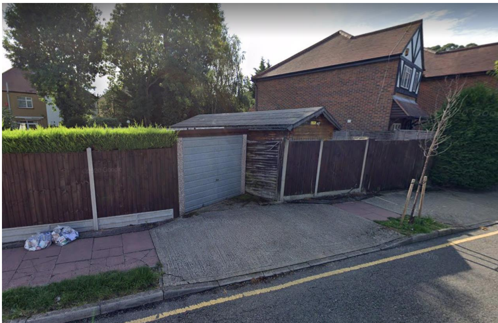
Figure 3.1 – Existing garage and dropped kerb
