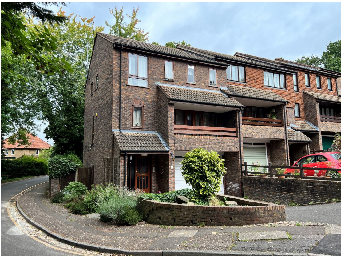
The dwelling on the adjacent corner to the south at No. 1 Ashbourne Square is positioned 1.5 metres away from the highway boundary at the closest point.
