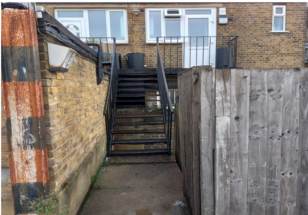
Photograph 6: Existing stair access to rear of first floor flats, Nos 72A and 73A
