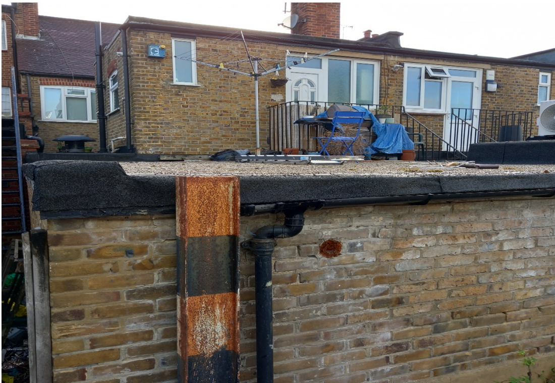
Photograph 4: The appeal property, from rear service road, showing flat roof of the ground floor unit which is, in part, used (in front of the railing) by the first floor flat.
