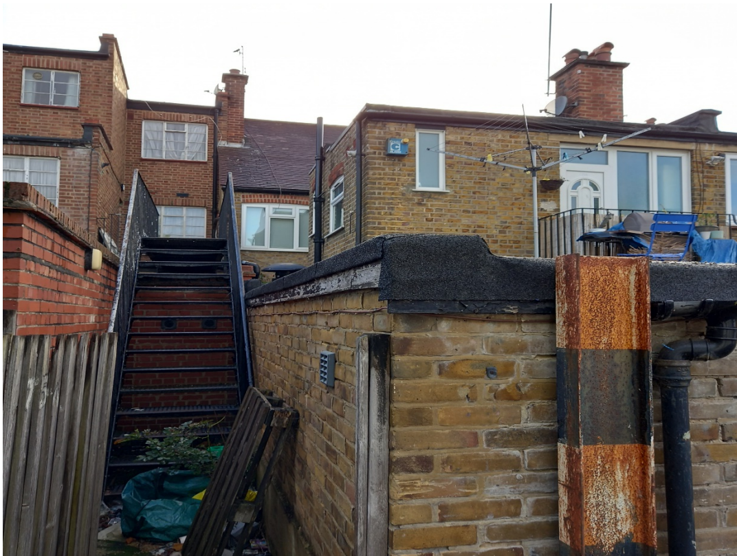
Photograph 5: Existing stair access to the flat above No 75. Appeal property on the right. Also showing rear roof slope of the appeal property, where a dormer extension is proposed.
