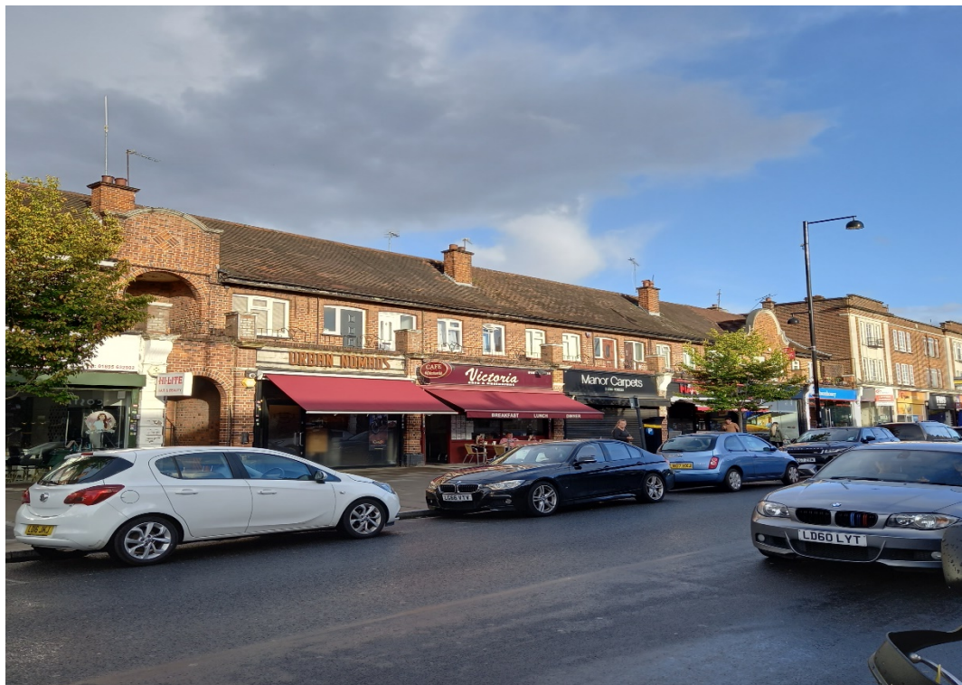
Photograph 2: The terrace, looking south from Nos 61 to 73 (appeal property), showing the change in scale beyond No 73 and the central (sole) entrance to the front access balcony.
