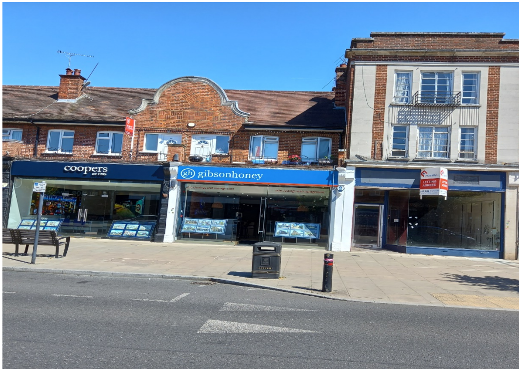
Photograph 1: The appeal property (centre) from the front, showing change in scale of neighbouring terrace. Front access balcony sits beyond the shop fascias and directly in front of the first floor windows.
