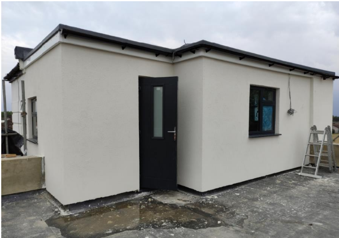
Existing access onto flat roof
