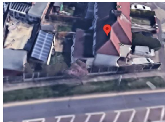
Solar Panels at Rear of No. 174 Yeading Lane
