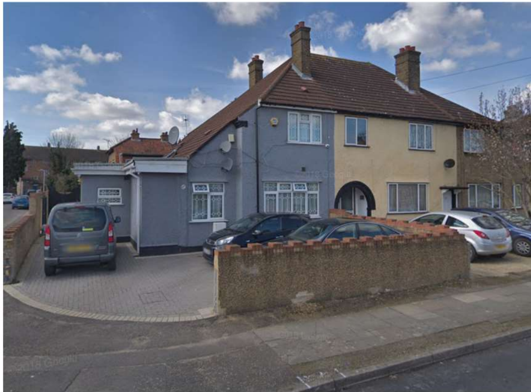
Figure 1: Front elevation of the appeal site
