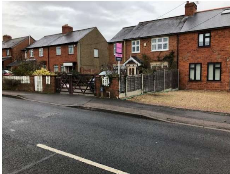
Walls, fencing and gates
