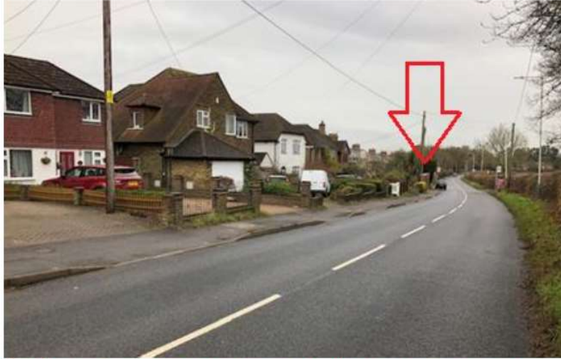
Wall, pillars and gate at 242 Northwood Road not conspicuous in street scene
