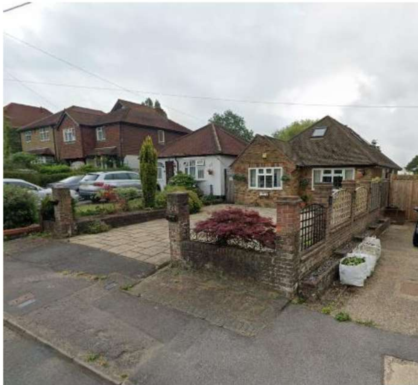
Walls, pillars, and railings
