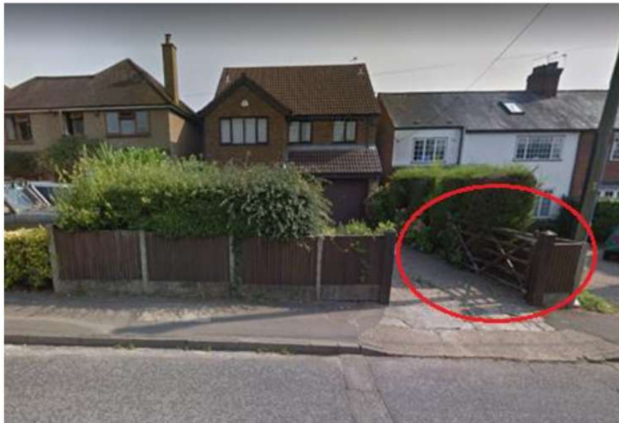
Five bar gate previously installed at the site (circled in red)
