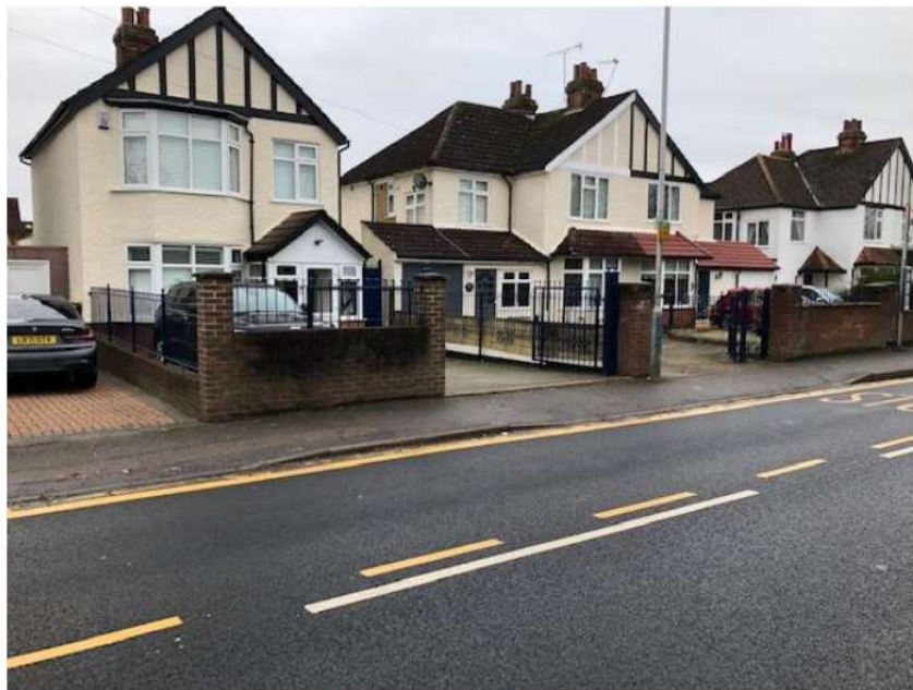
Walls, pillars, and railings
