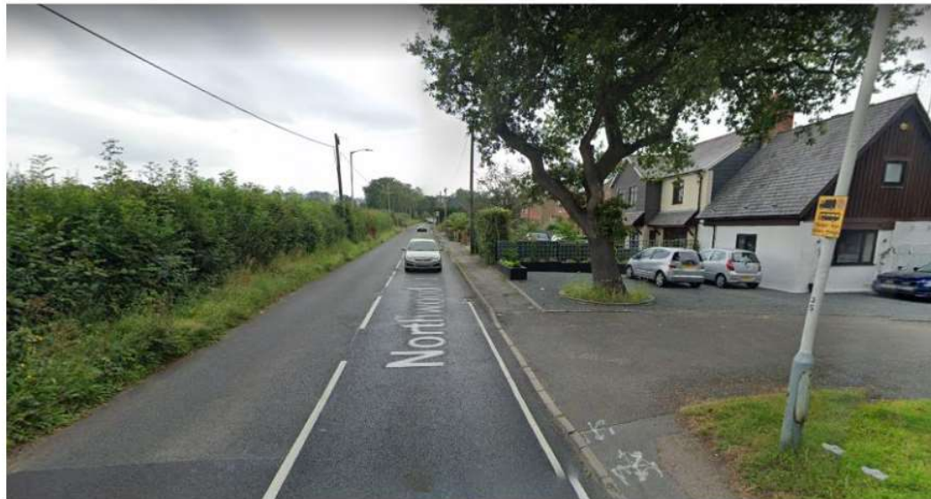
View north along Northwood Road
