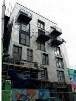
Boilerhouse, nearing completion
