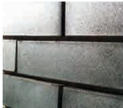
Boilerhouse brick cladding
