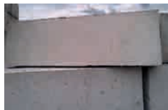
precast concrete (lintels to Block B)
