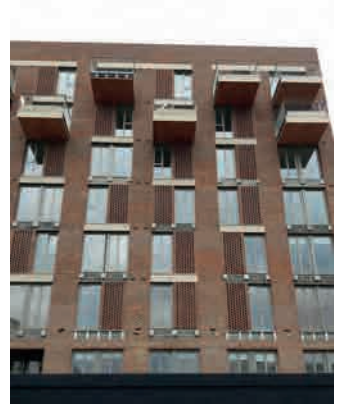
Material Store, nearing completion
