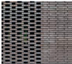
Material Store brick
