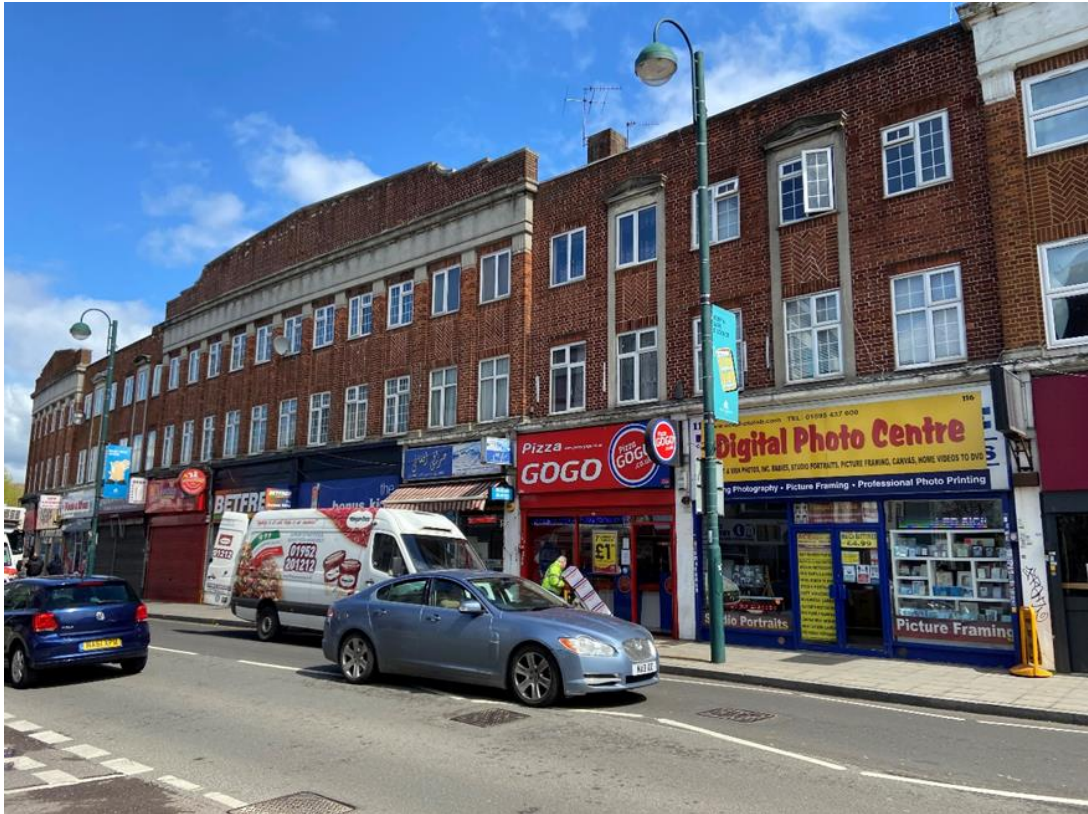
Image 7: Three storey terrace at Nos. 112-134 High Street with residential accommodation at upper floor levels within Yiewsley District Centre
