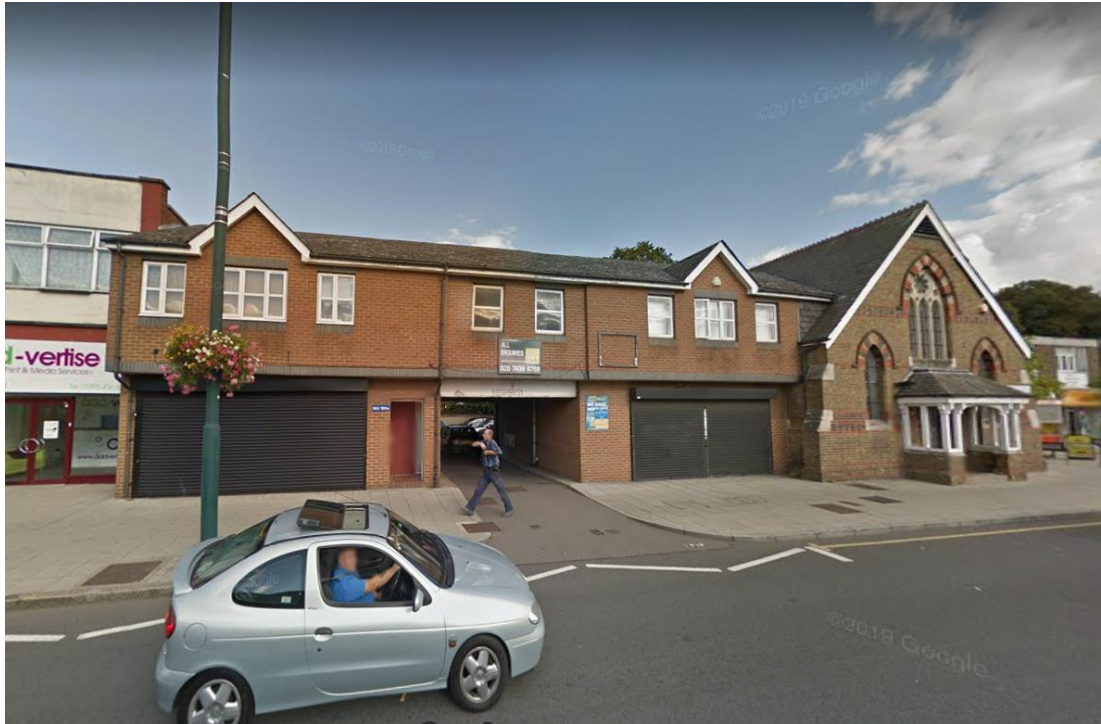
Image 3: Image of the wider parade facing south east demonstrating clear variation in both the height and design of buildings present
