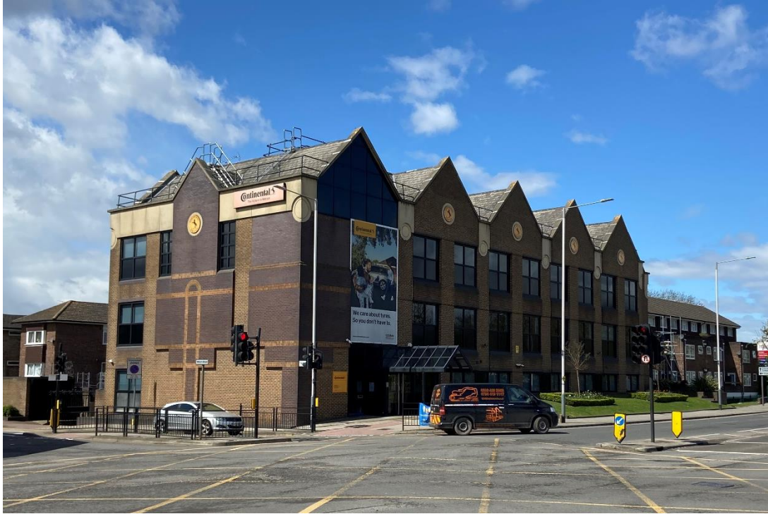
Image 9: Three storey office development known as Continental House that bookends the northern side of Yiewsley District Centre
