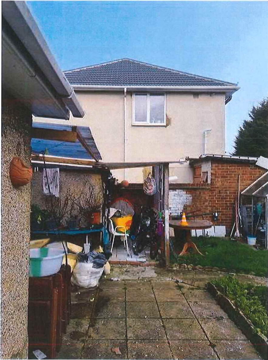
Side elevation of no. 11 Skipton Drive from appeal site patio area
