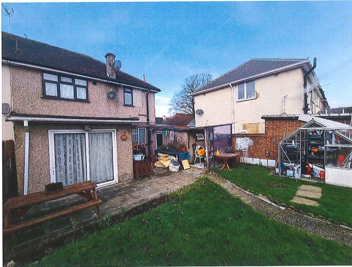
Boundary with adjoining neighbour no. 11 Skipton Drive
