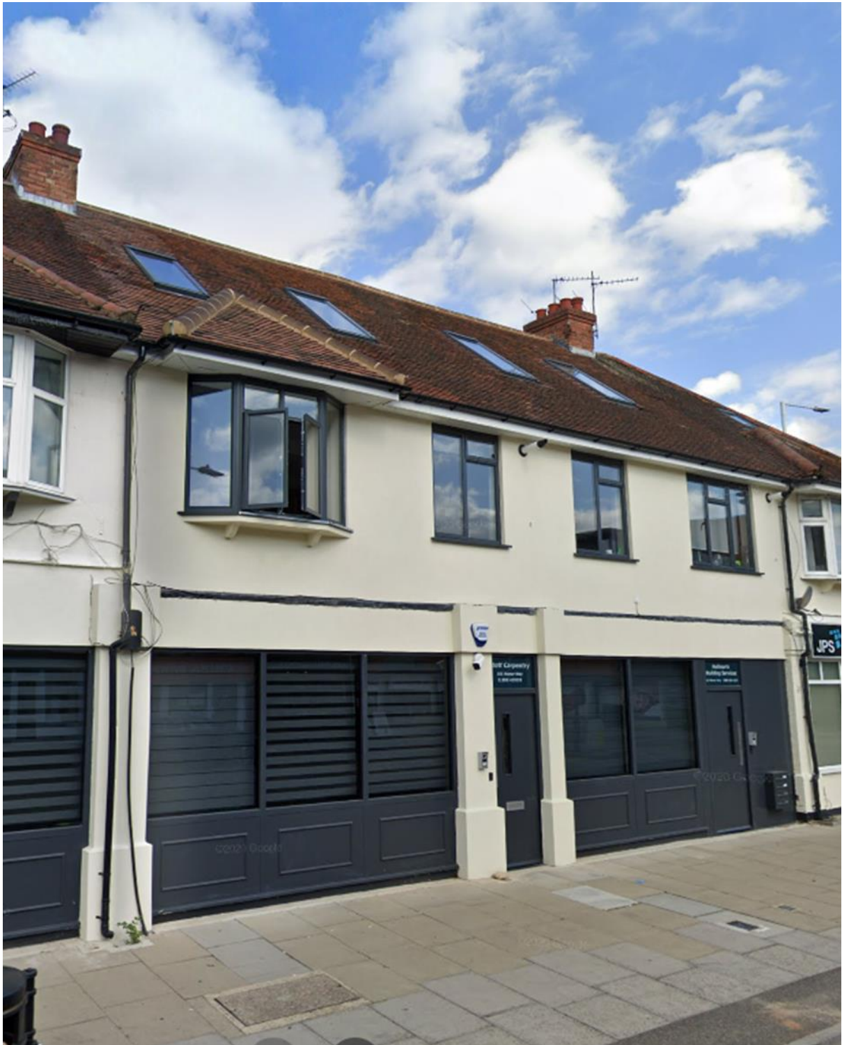
Image of rooflights on Manor Way.
