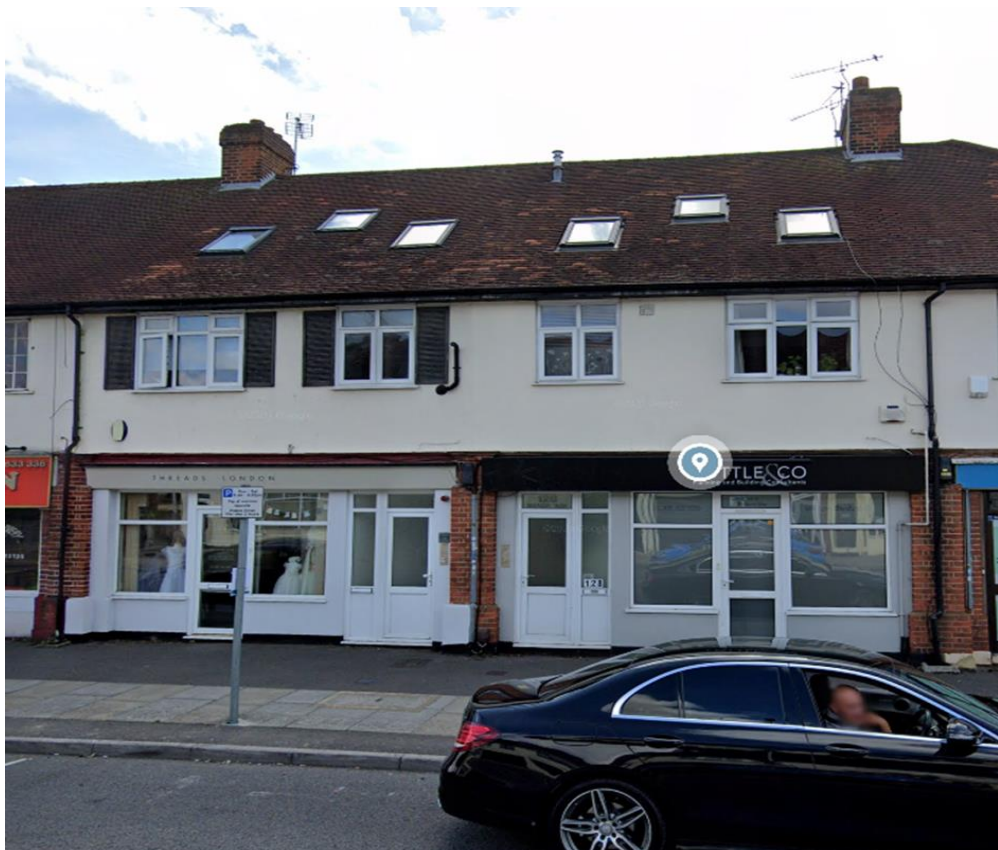
Image of Rooflights on Manor Way
