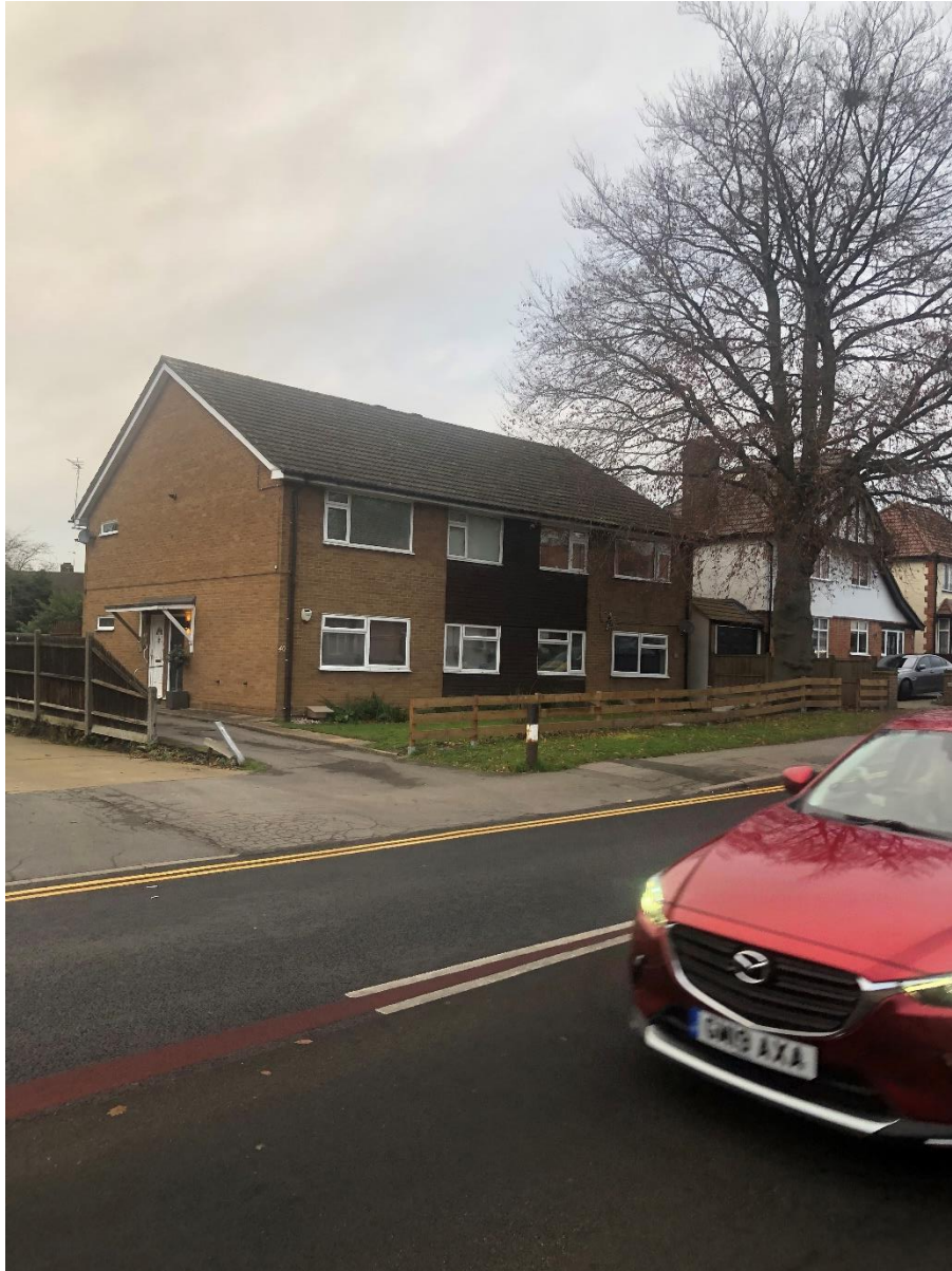
View of site across Windmill Hill heading northbound
