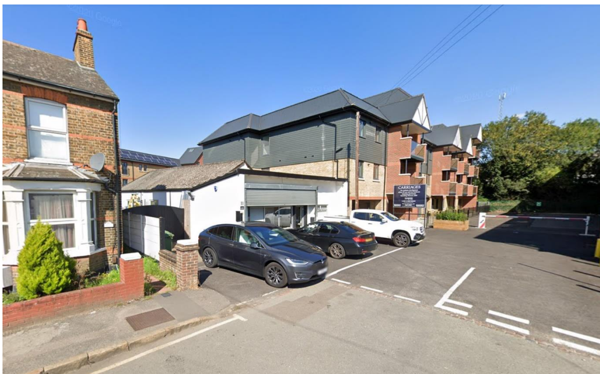
No.1 Wariwck Road (left), application site (middle), Pullman Court (right)
