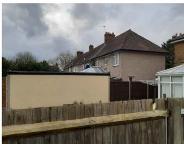
REAR OF No.14 EXTENSION
