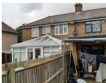
REAR OF No.16 EXTENSION
