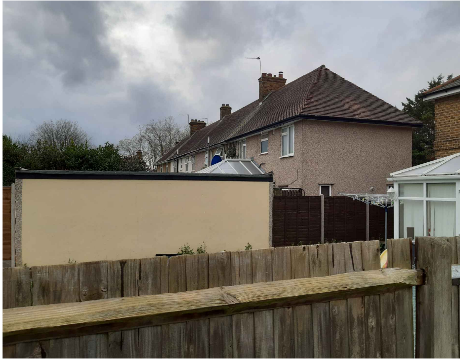
REAR OF No.14 EXTENSION
