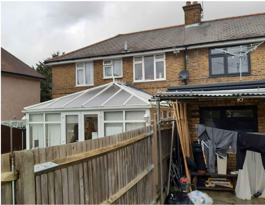
REAR OF No.16 EXTENSION
