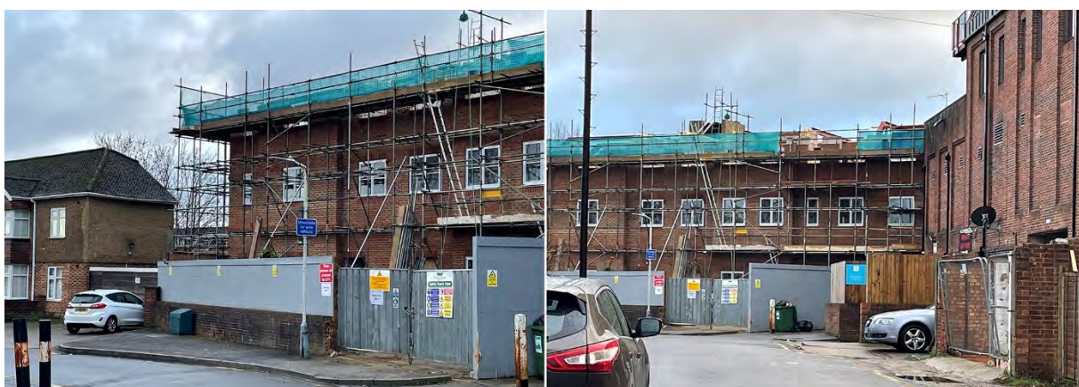
New development at rear of 53-55 Joel Street on Ferndown to second floor window level – December 2021
