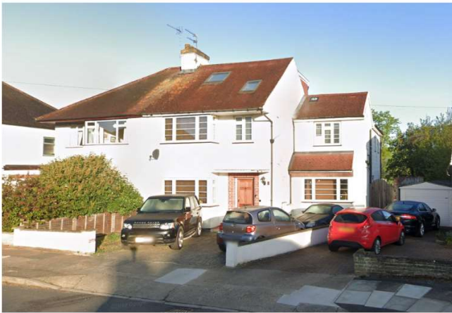
Figure 1 – Front view of existing dwelling
