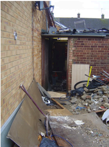
Entrance of the garage accessed from rear garden
