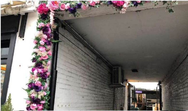
Undercroft access to site from High Street.
