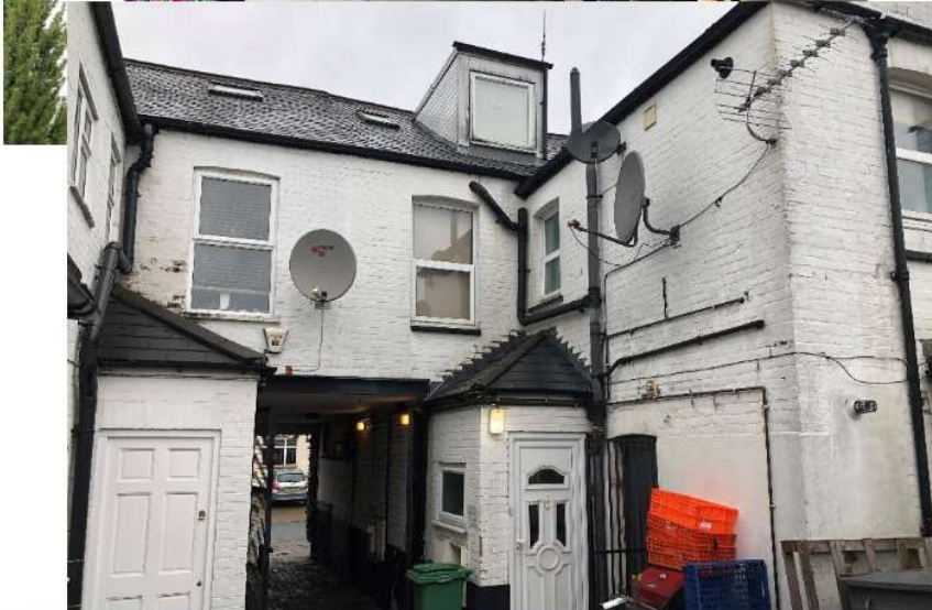
Left: Looking back at existing window arrangement
