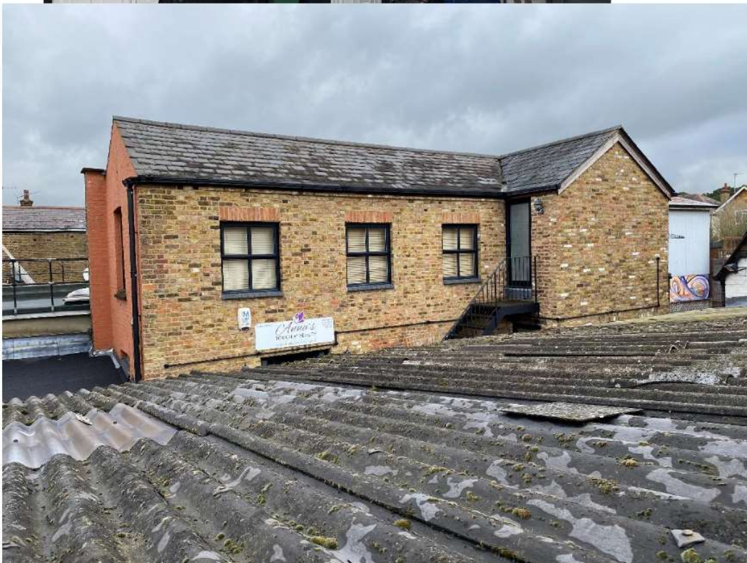
Above : Existing building at no. 20 High Street
