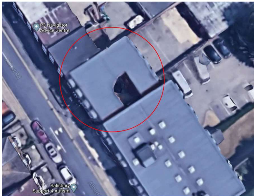
PHOTO 1: SHOWING REAR OF THE APPLICATION SITE
