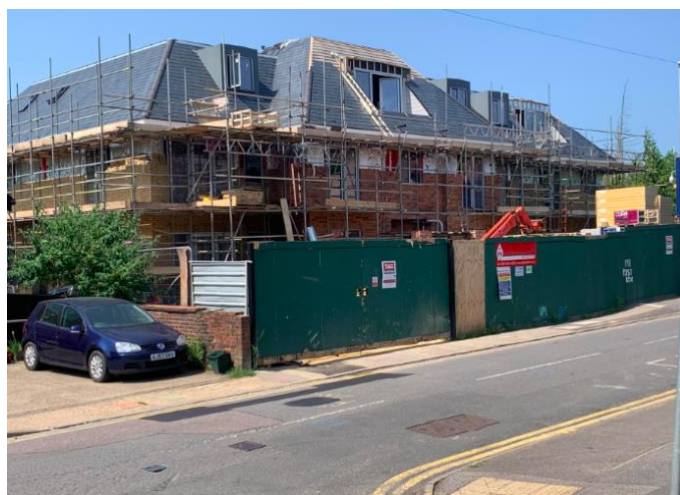
Development of the former Abrook Arms PH
