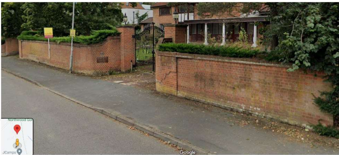
Byworth house 20 Linksway– high brick walls and high piers and gates
