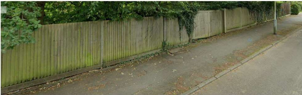
3A Linksway – closed high boarded fence panels with timber gates running the length of the front giving an austere, isolated feel
