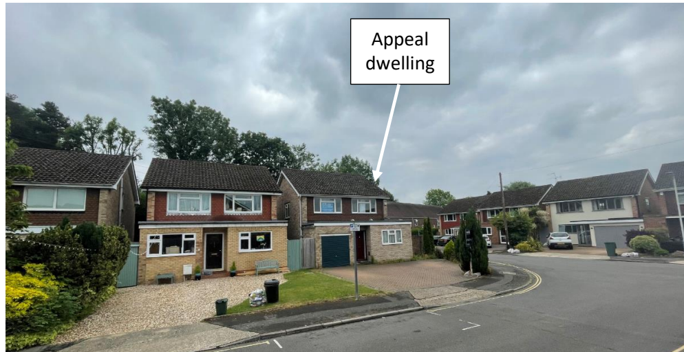
Appeal site and dwellings to the south east side of The Mallows
