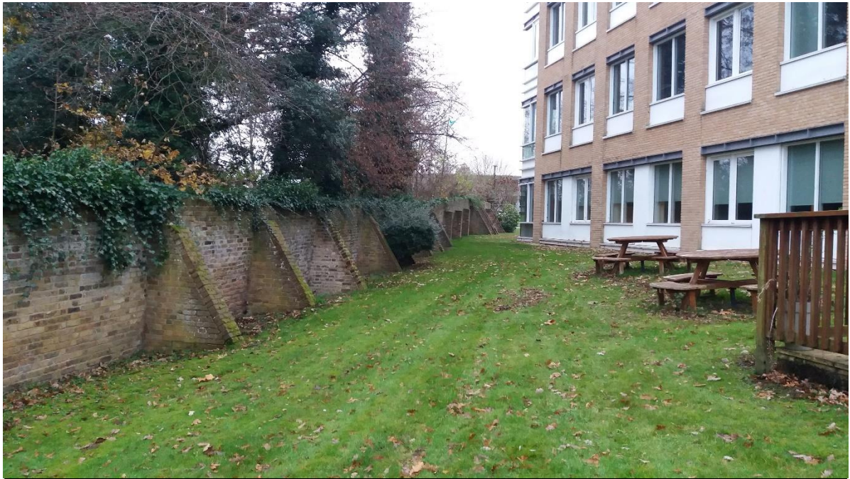
Figure 2.0. – Retained section of former walled garden brick walls to the east of HPN Date: 15.12.2021
