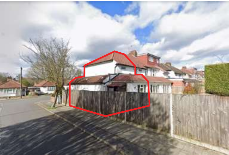
(above) Side extension to 31 Hazelwood Drive viewed from the rear
