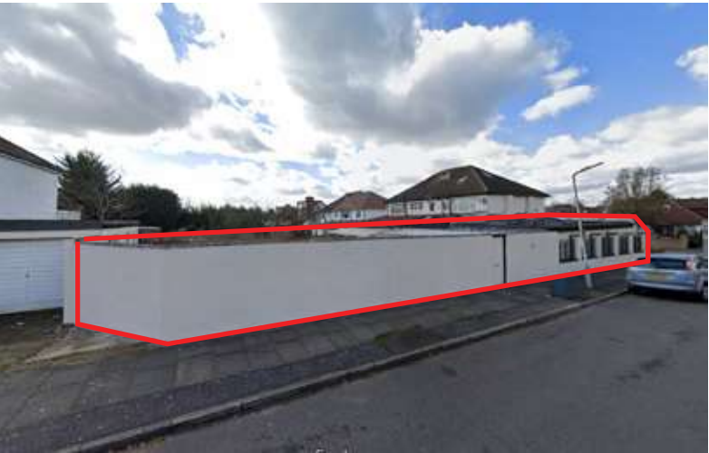
(above) Side extension to 9 Hazelwood Drive viewed from the rear
