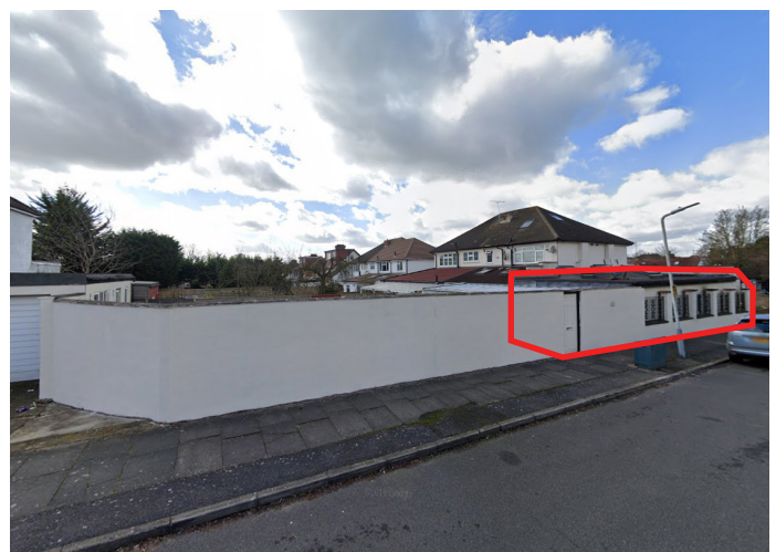
(above) Side extension to 9 Hazelwood Drive viewed from the rear
