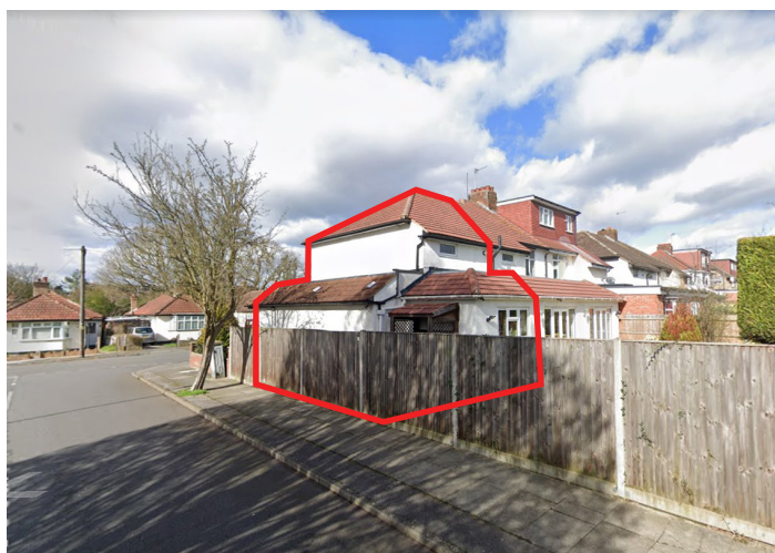
(above) Side extension to 31 Hazelwood Drive viewed from the rear
