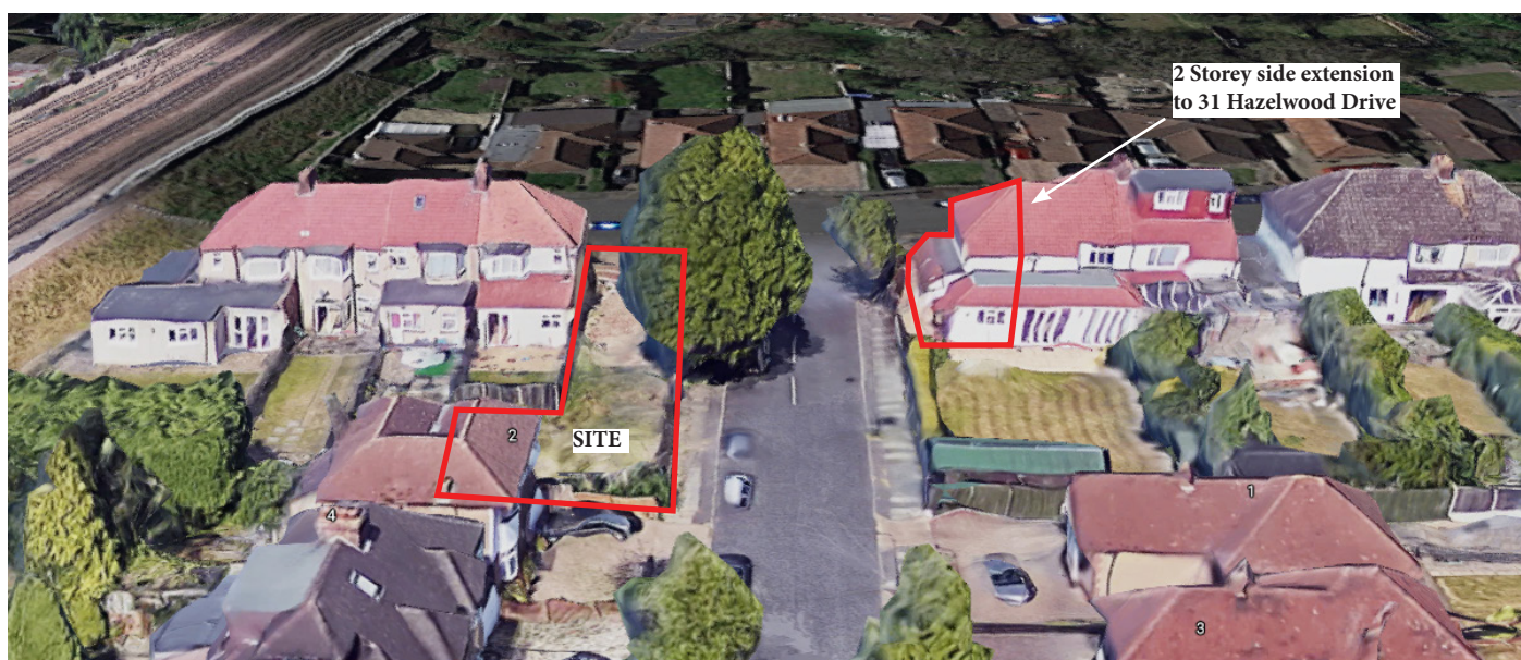
(above) Side extension to 31 Hazelwood Drive viewed from above
