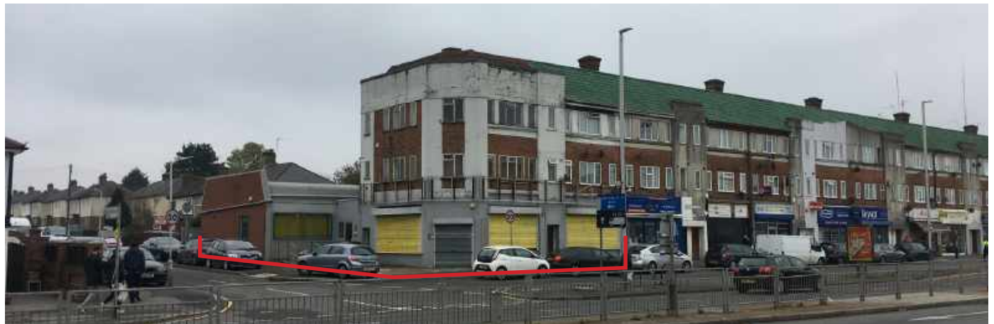
Streetview of site
