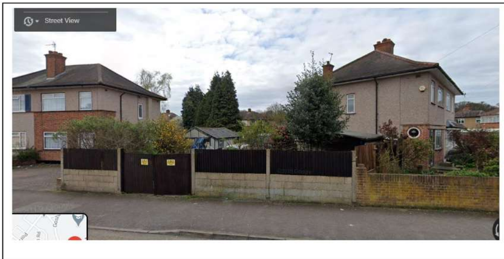
Figure 1 Open gap between 1 Adelphi Crescent and 3 Adelphi Crescent
