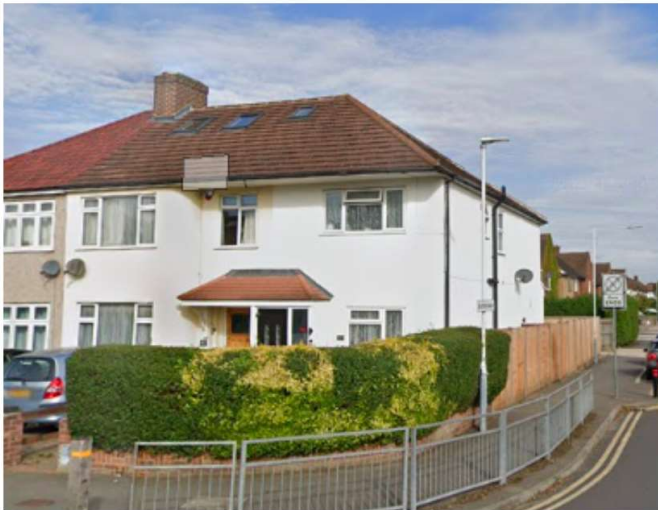
162a Long Drive, Ruislip, HA4 0HR
