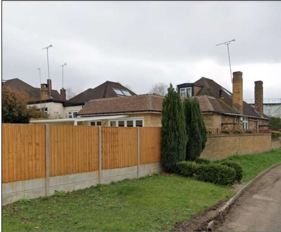
Figure 2: Image of the rear of the appeal property.
