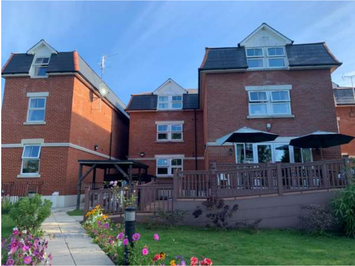
Photograph: Rear of 34-38 Chester Road, September 2019
