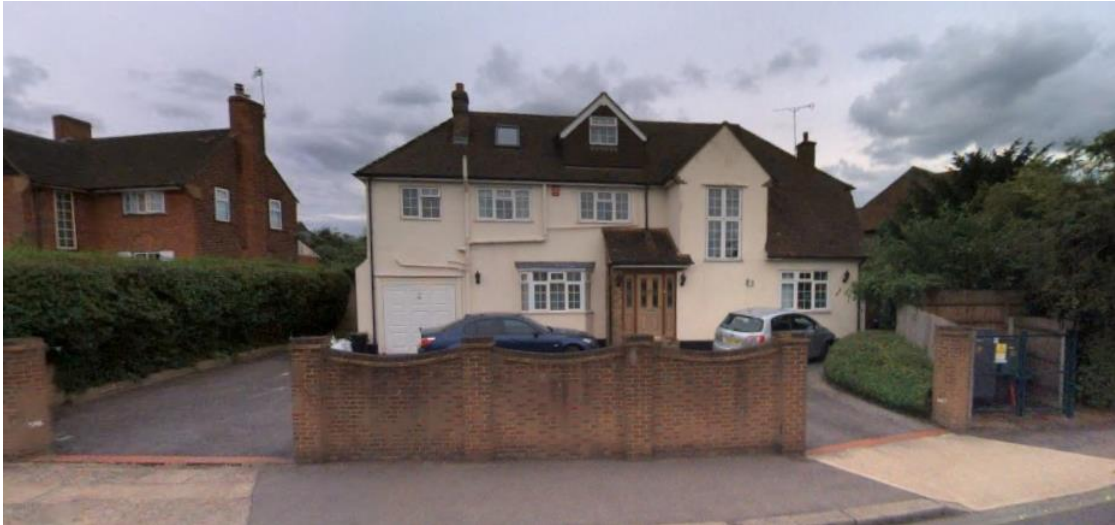
No. 51 Ickenham Road
