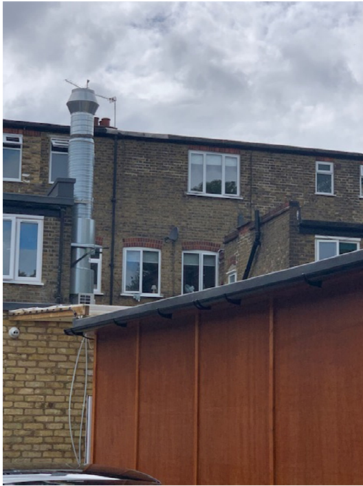
figs. 3, 4 new flue and cooling equipment installed on the roof of the new extension, in the same location as the pre- existing flue
