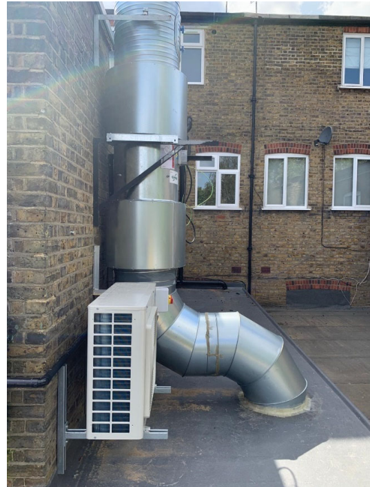
figs. 3, 4 new flue and cooling equipment installed on the roof of the new extension, in the same location as the pre- existing flue
