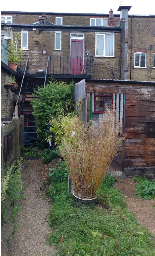
fig. 1 The pre- existing condition at the rear of the building, showing the kitchen flue attached to the flank wall of the existing rear extension
