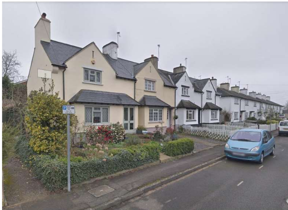
View of Cordingley Road showing the original terraces to the east side of the road
