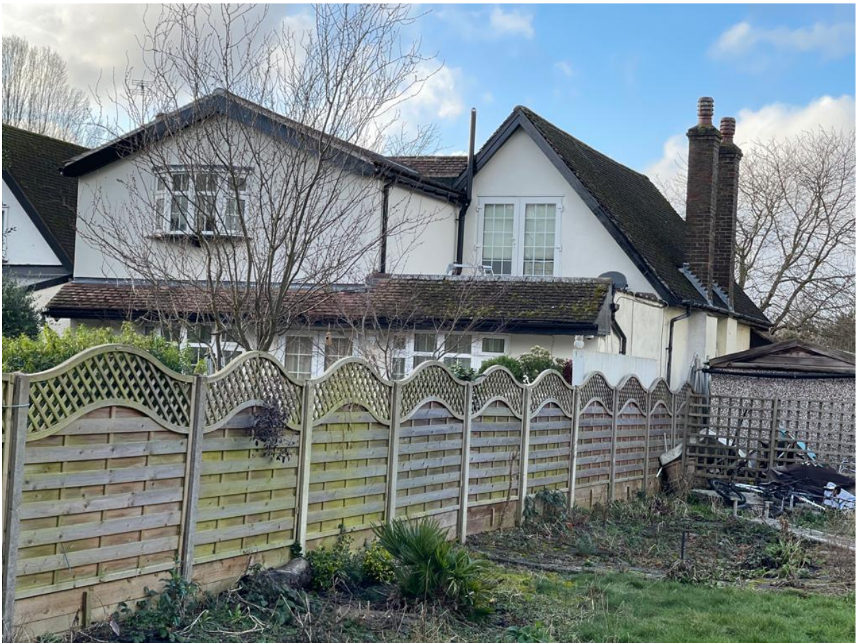
The 2-storey rear extensions at number 21 with its catslide roof housing 2 protruding chimneys
