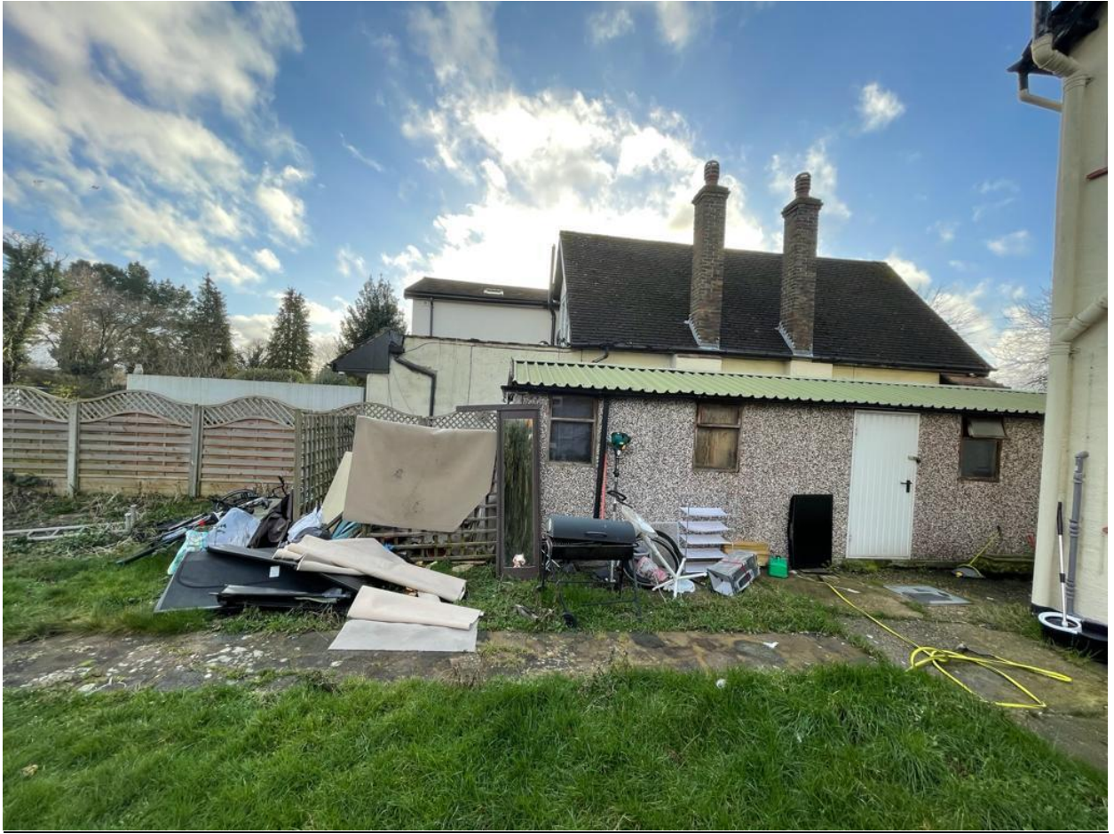
Appeal site juxtaposed with number 21 and its substantial rear outrigger extensions
