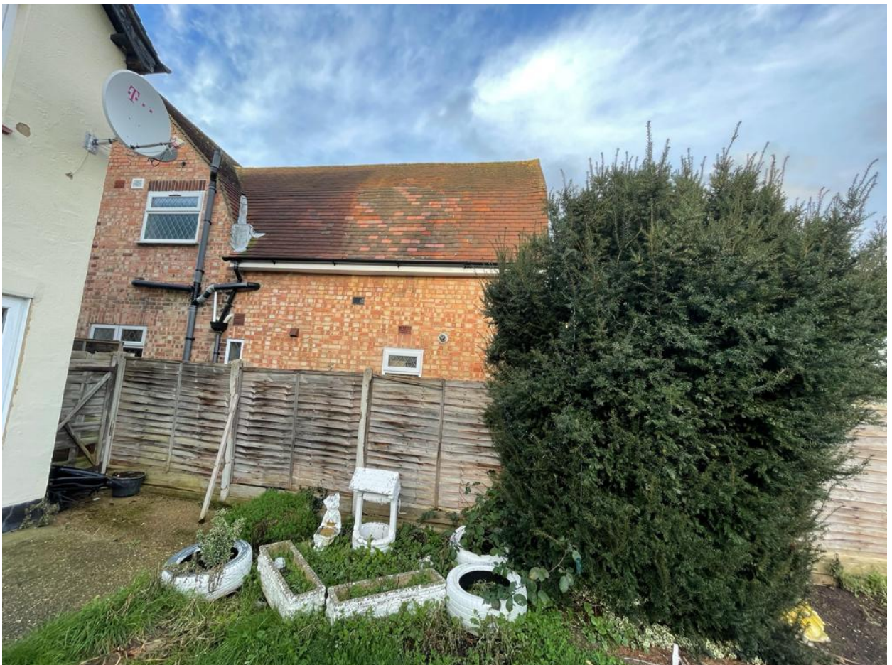
Appeal site juxtaposed with number 17 and its two storey outrigger extensions
