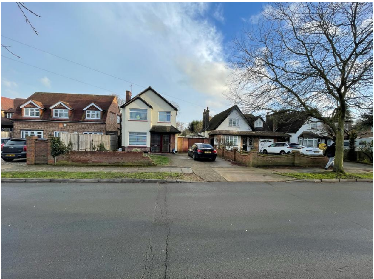
Street view presently Lawn Avenue elevation with number 17 on the left and 21 on the right
