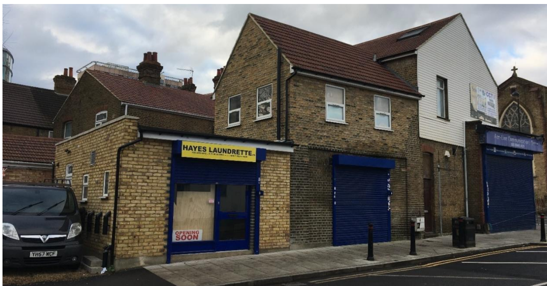
North elevation of 63 Station Road (looking south) - showing the single storey rear extension approved under application ref: 18175/APP/2017/2180
