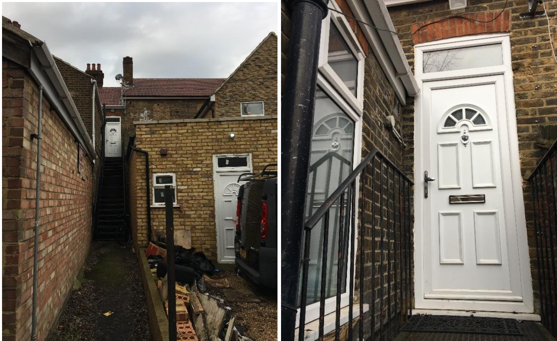
Rear alleyway, obscured window and entrance door between 65-67 Station Road and 67A Station Road
