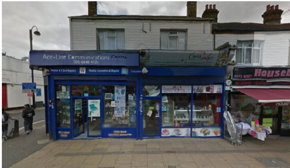
NOS. 63 & 65 STATION RD UB3 4BG-STATION RD(WEST) ELEVATION
