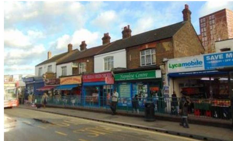
NOS. 63 & 65 STATION RD UB3 4BG-STATION RD PARADE(WEST)
